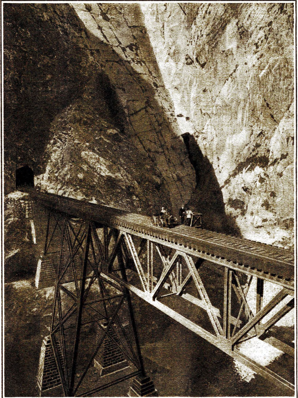
THIS TRESTLE IS 13,500 FEET IN THE AIR. IT IS ONE OF THE ENGINEERING FEATS ON THE OROYA RAILROAD, FROM OROYA TO CALLAO, PERU. ON THIS ROAD THERE ARE 67 TUNNELS, 65 TRESTLES, AND 17 SWITCHBACKS. TICLIS, AT AN ALTITUDE OF 16,000 FEET, IS THE HIGHEST RAILROAD STATION IN THE WORLD.
